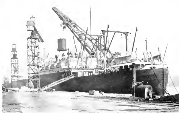
View of the outfitting dock, Mare Island Navy Yard, showing one of hammer-head cranes on the pier and the 150-ton floating crane outboard.
